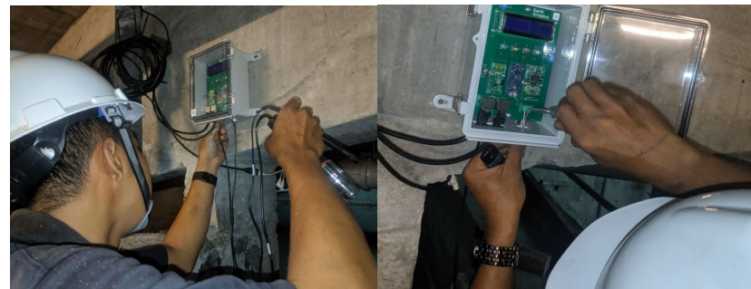
Sensor control unit and sensor connection/power supply connection
