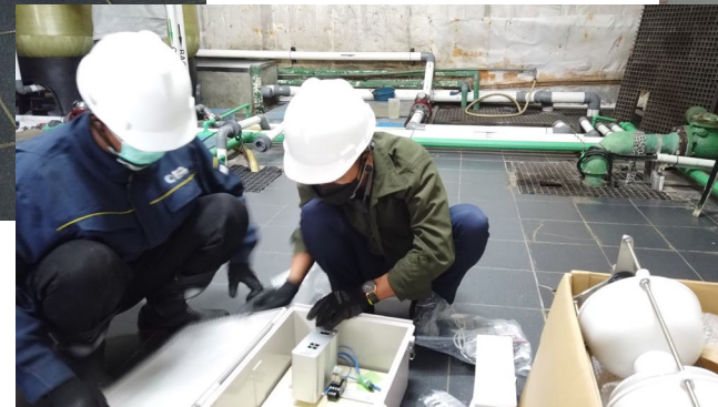
Installation of IoT monitoring system control panel
